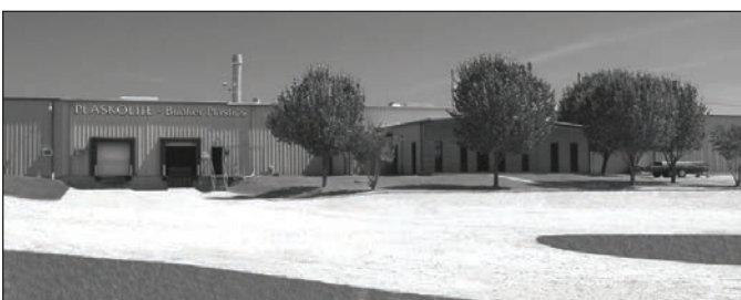
Grand Saline, Texas, USA Manufacturing and Distribution
