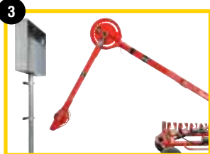
Align with conduit, properly adjust booms
