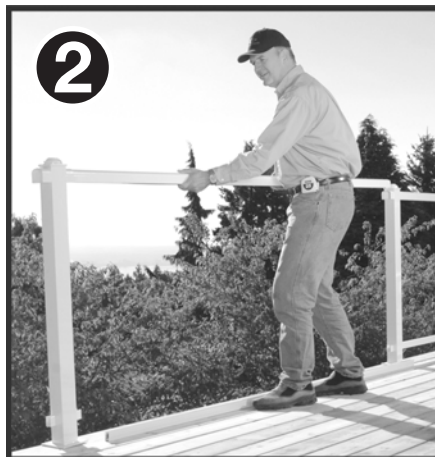
STEP ② INSTALL RAILS
