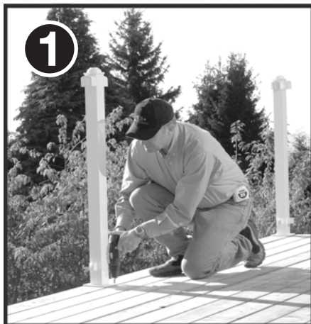
STEP ① INSTALL POSTS
