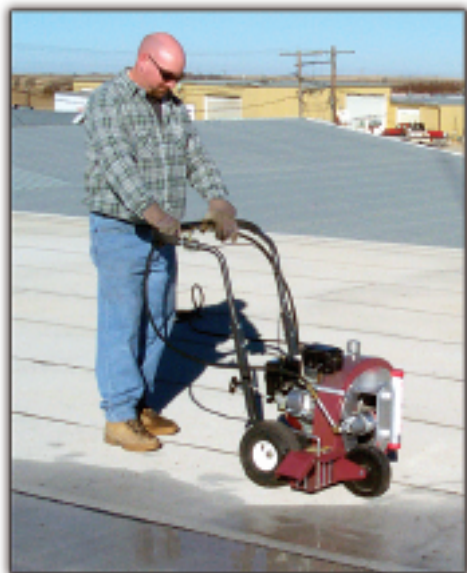
Red Dragon Roof Dryers combine high heat and a powerful blower to dry roofs quickly.
