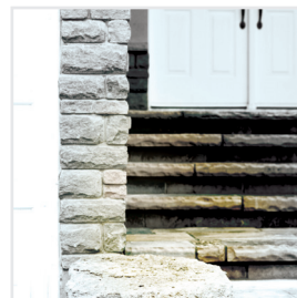
Fills in cracks in concrete
