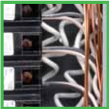
Pigtail Neutral Connections
