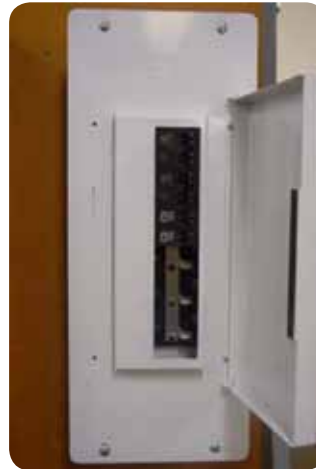
Step #3 Install New HFLCI
