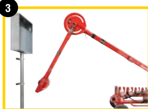
3 Align with conduit, properly adjust booms
