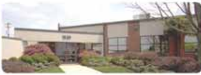
Hickory, North Carolina
