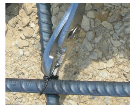
Typical TW installation
